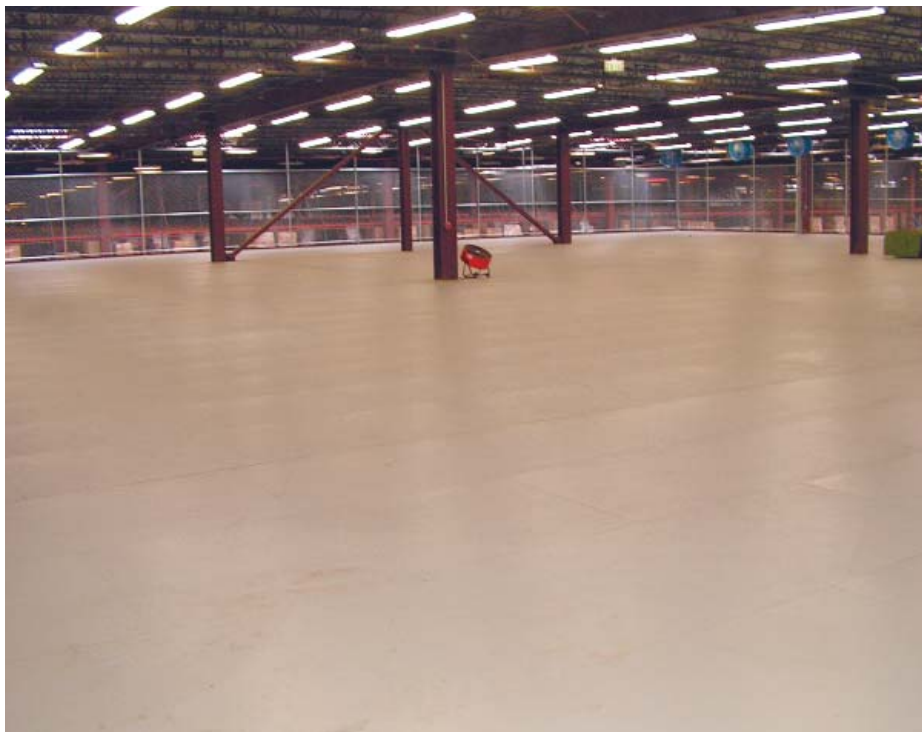
ResinDek® panels installed on new elevated platform
