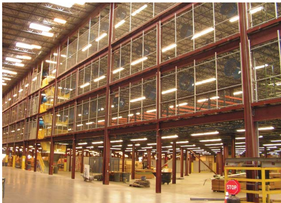
Concrete Platforms require lots of steel
