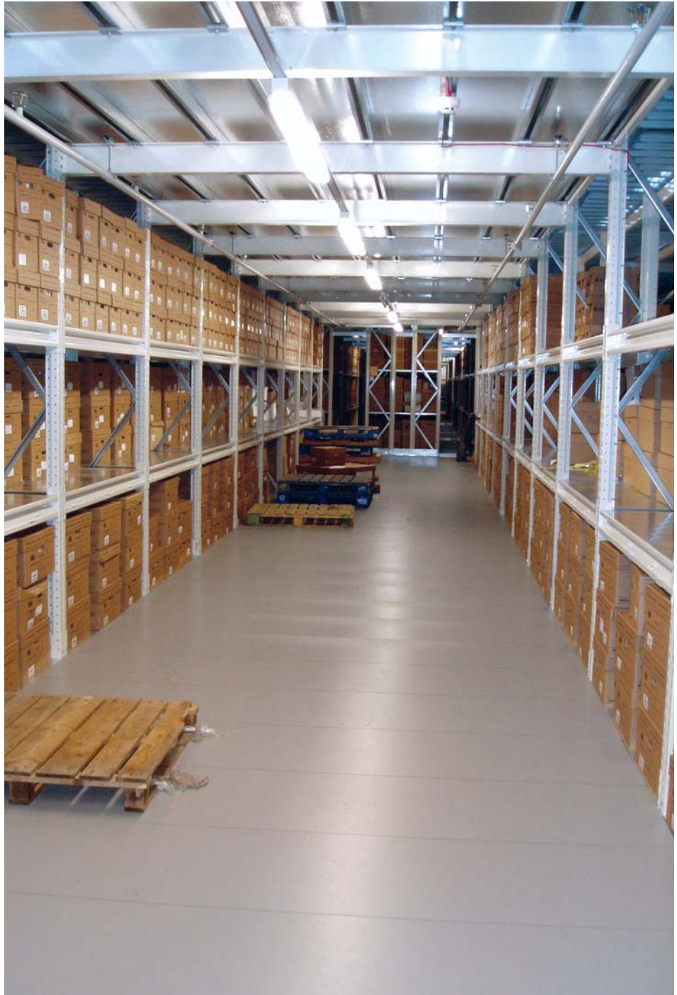
Iron Mountain ® in Belvedere, UK with ResinDek Xspan installed for rigorous loads of 1,000 kilograms 100 times a day
