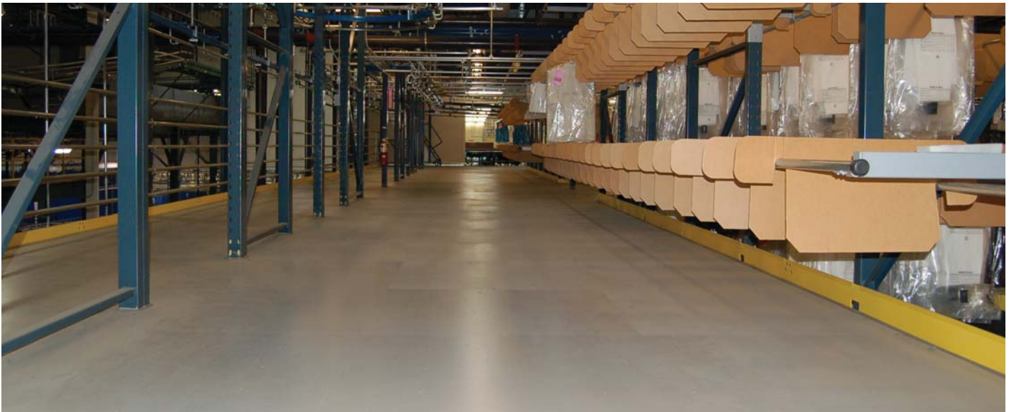
Polo Ralph Lauren facility with ResinDek products installed
