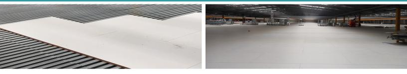
A project located in Manchester, U.K. had a three level mezzanine with 220,000 sqft per level. The flooring system that was selected was 3/4" ResinDek HD with the TriGard<sup>®</sup> ESD finish and corrugated steel decking. During the final walk through, the Main Contractor made the following comments:
