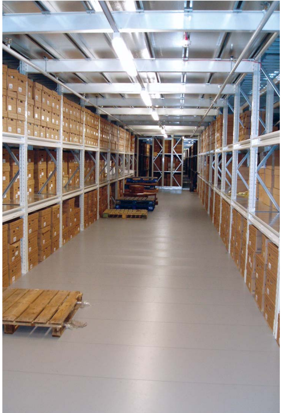
Iron Mountain ® in Belvedere, UK with ResinDek Xspan installed for rigorous loads of 1,000 kilograms 100 times a day
