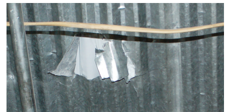
Attempted repairs beneath the mezzanine to block debris from falling through.
