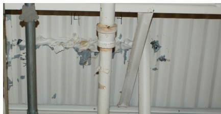
Attempted repairs beneath the mezzanine to block debris from falling through.
