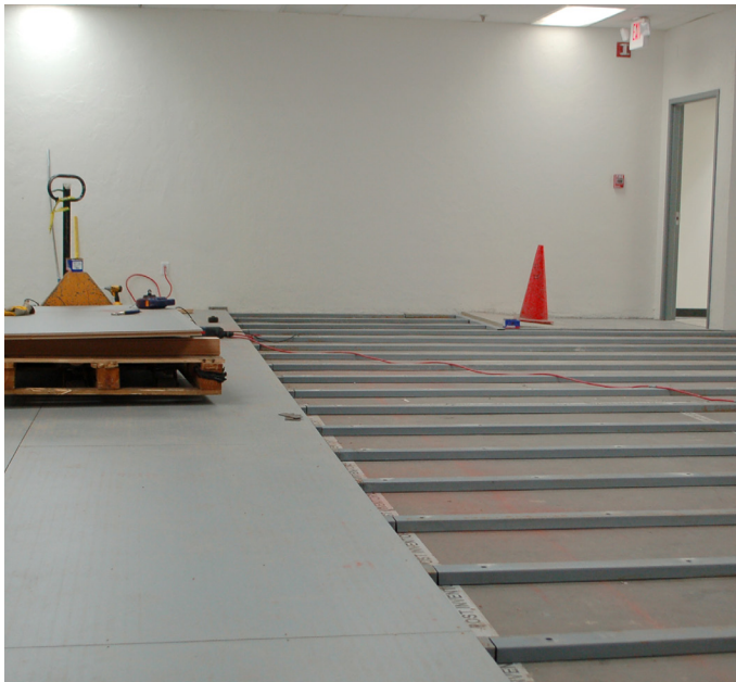
Installation of ResinDek and steel sleepers over damaged concrete.
