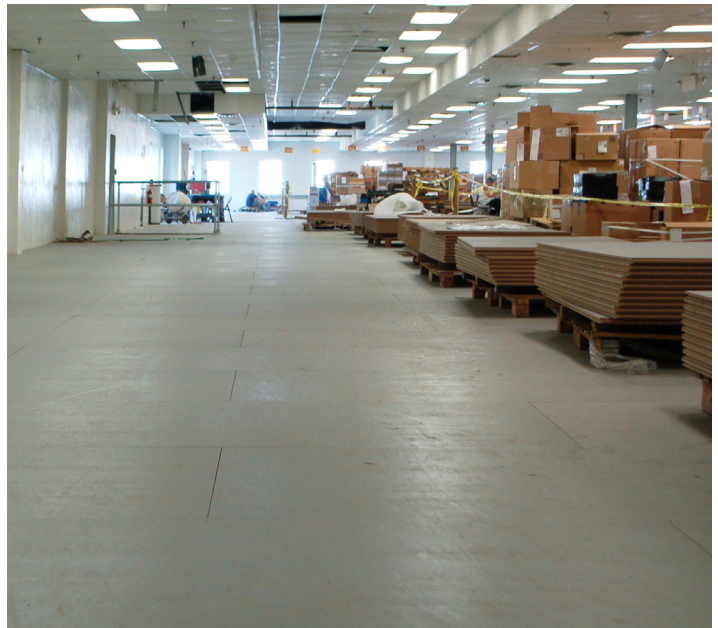
ResinDek installed and loads moving easily.
