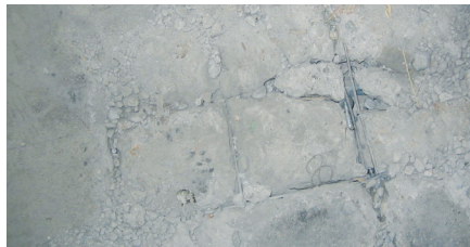
Concrete mezzanine flooring with significant damage prior to ResinDek.
