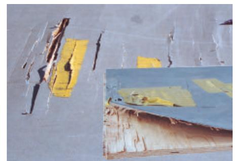
Extensive substrate failures and "alligator skin cracks" were evident throughout this job site before the poly-deck was replaced.
