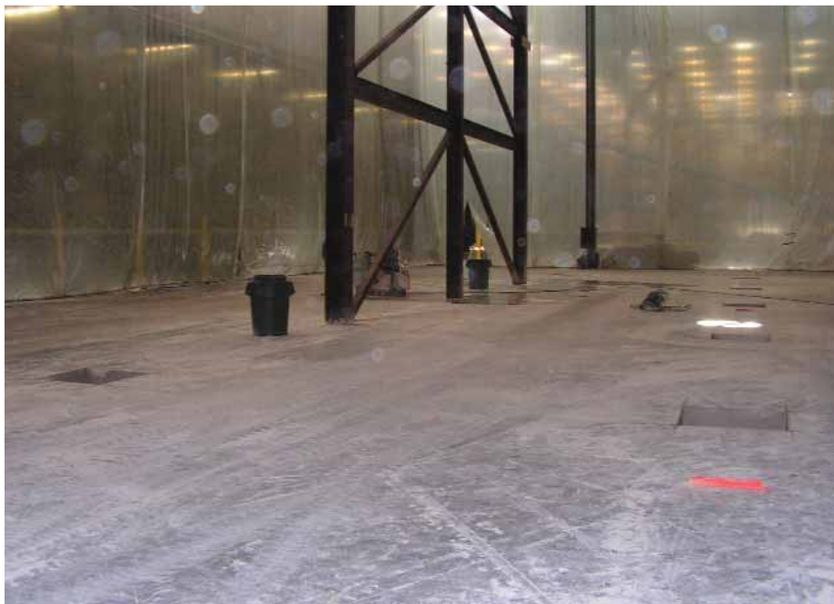
Prepping for re-engineered ResinDek® Mezzanine at Sporting Goods Facility in Texas
