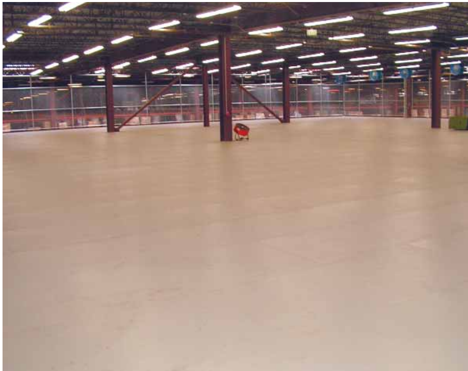
ResinDek® panels installed on new elevated platform
