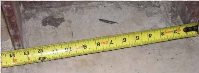
Heavy concrete structure requires massive footings and 14" columns
