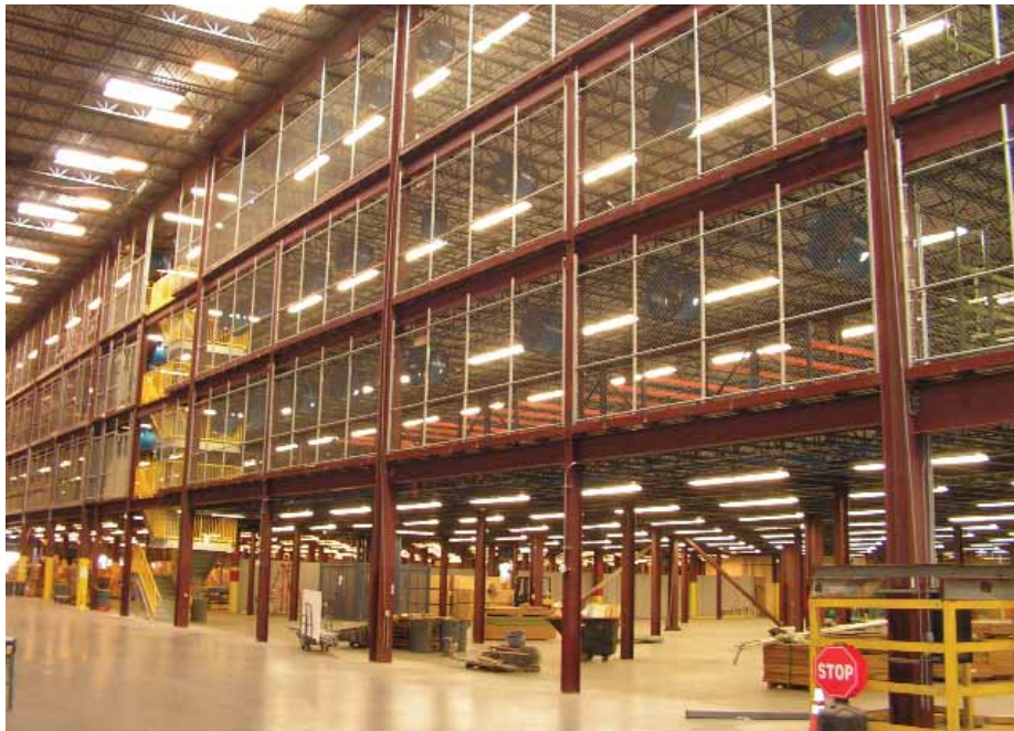
Concrete Platforms require lots of steel
