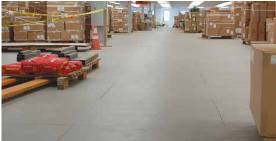
New ResinDek® panels installed
