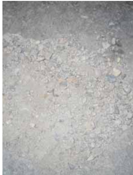
Concrete mezzanine flooring with significant damage prior to ResinDek
