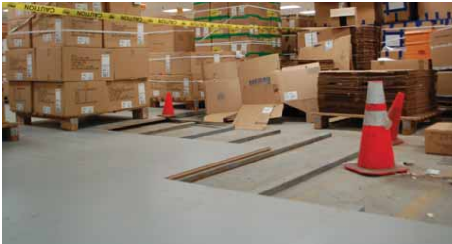
Installation of ResinDek and steel sleepers over damaged concrete
