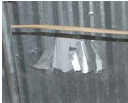
Attempted repairs beneath the mezzanine to block debris from falling through
